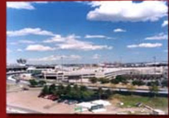
Continental Airlines Terminal C Parking Garage Newark, NJ
