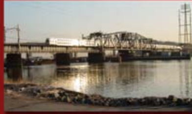
Portal Bridge Capacity Enhancement Hudson County, NJ
