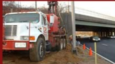
Interstate 295 and Route 38 Improvement Burlington County, NJ
