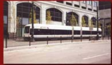
Hudson-Bergen Light Rail Transit System Hudson and Bergen Counties, NJ
